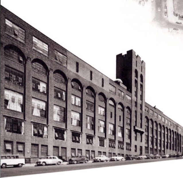
A wing of the New York Plant
